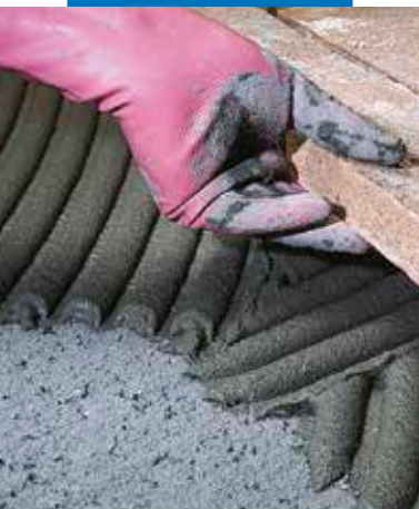
Installation of hand made terracotta on an uneven substrate
