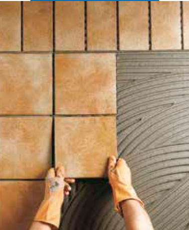
External installation of klinker tiles
