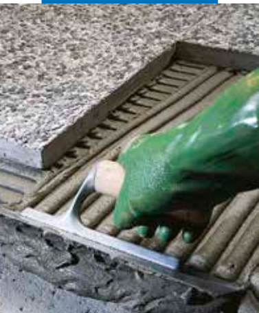
External installation of relief terrazzo "graniglie" tiles
